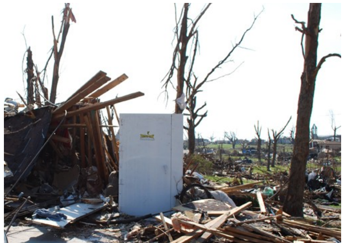
This In-residence Safe Room, (manufactured by a NSSA member) located in a garage protected two people (Joplin, MO).
